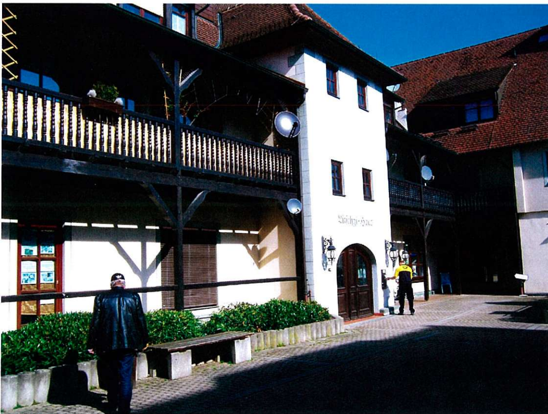
Basler Straße 7, 9, 10, 12 (Litschgi-Haus, Innenhof)
